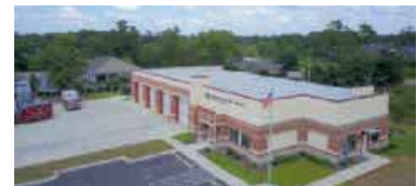
Horry County University Fire Station
