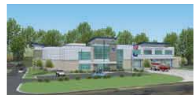
North Myrtle Beach Emergency Operations Center
