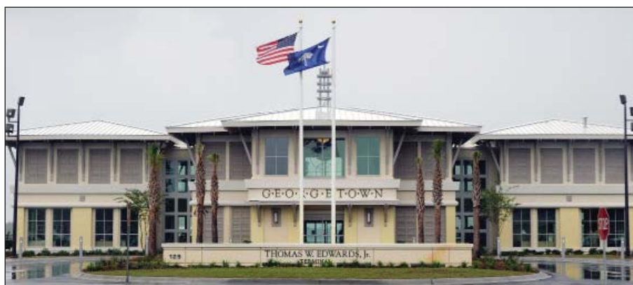
Georgetown County recently opened the Thomas W. Edwards, Jr. Terminal at Georgetown County Airport. The Georgetown County Airport Commission plays an integral role in making improvements to the airport, which receives about 24,000 aircraft per year.
