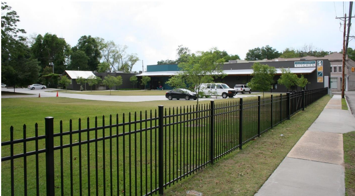
Today – The improved approach view from Wichman Street showing the completed Commercial Kitchen including parking, loading bays & fresh new landscaping across the
